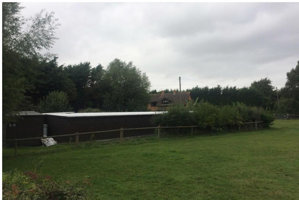
Figure 1. View of existing cattery on site
