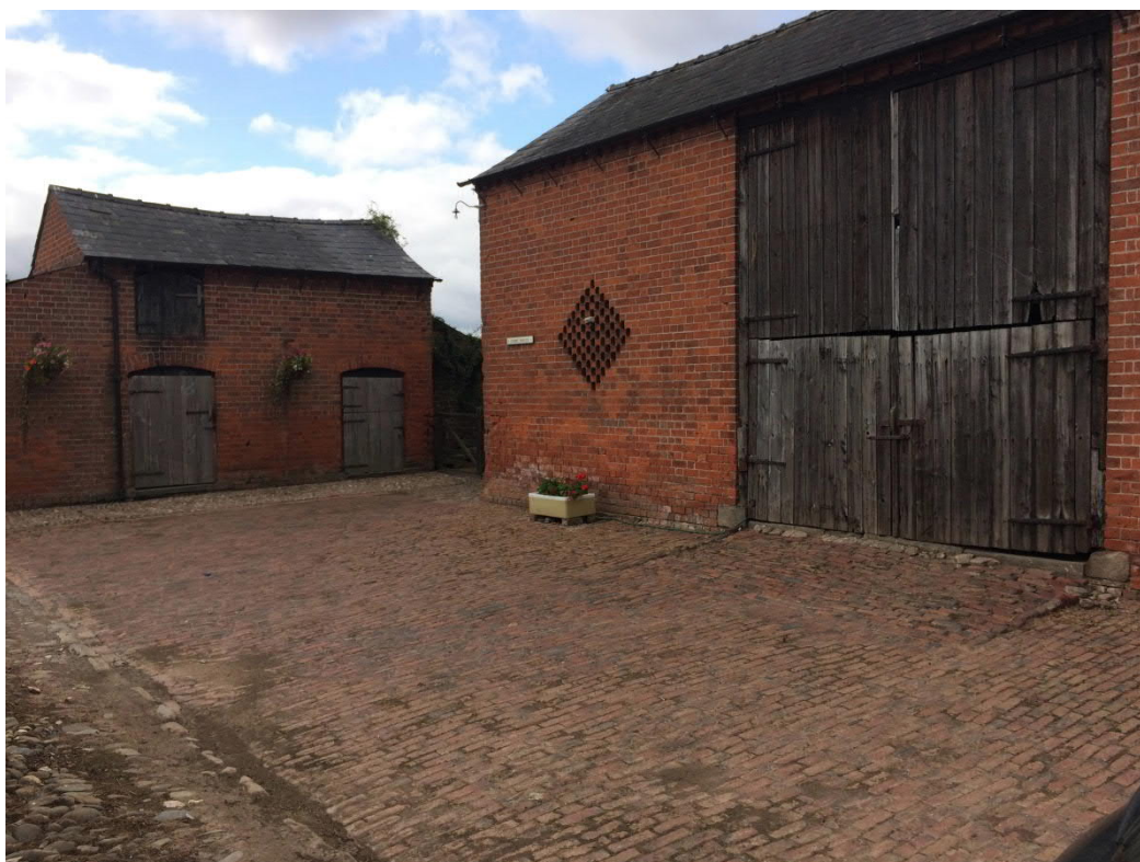
Figure 20. The barn proposed for conversion which makes up Site 16
